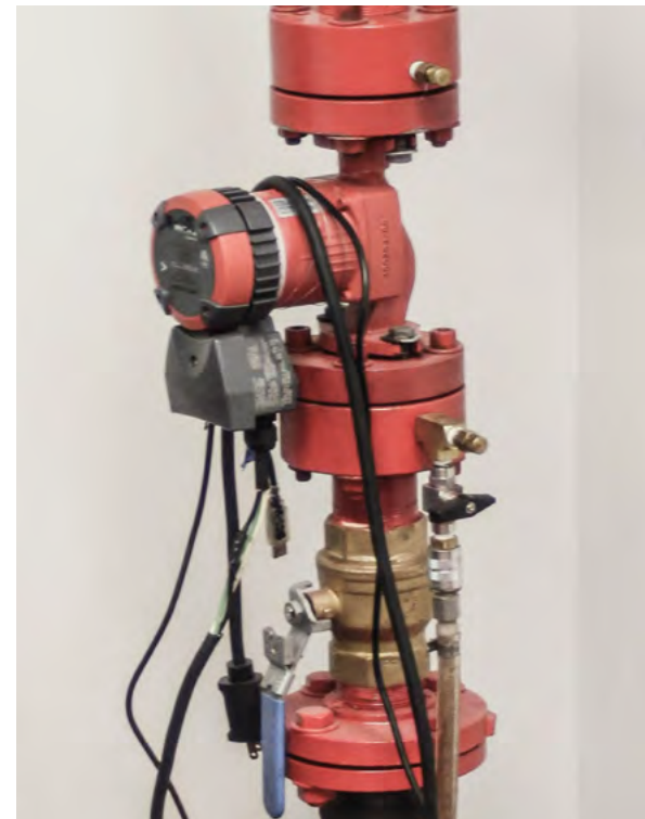
A1 circulator installed
